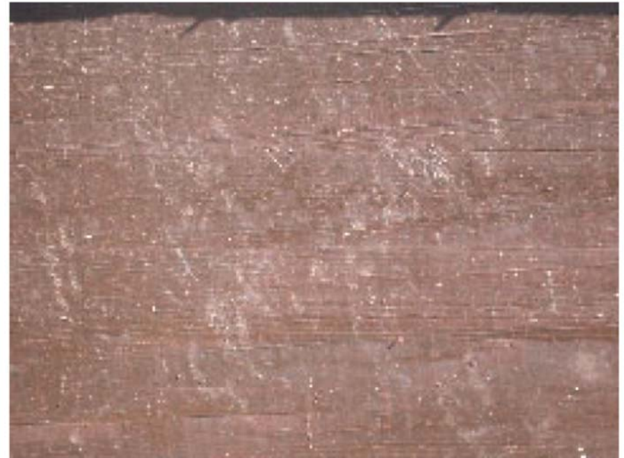
Photo 17: Detail view of gluelam beam
