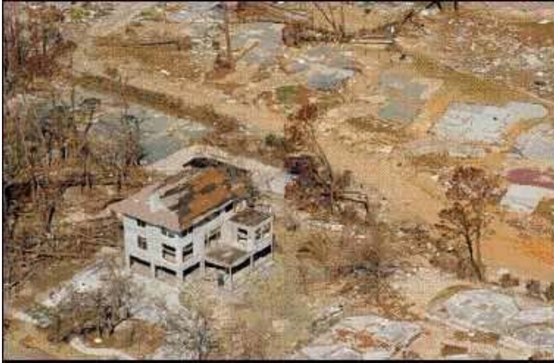
Concrete house left standing after Hurricane Katrina
