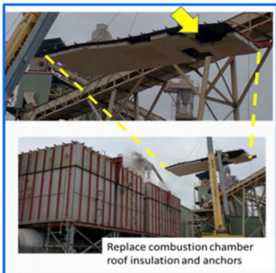
Insulation anchor failure with 304 SS RTO
